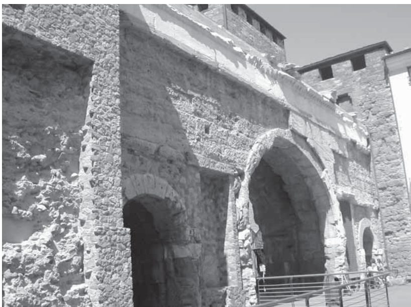
Fig. 1 – Eastern facade of Porta Praetoria, showing the cover with grey marble slabs and white marble cornice.
