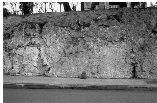
Fig. 15 – Tre Torri Hotel. Walls with evident traces of ancient working on typical structure of megabreccia.
