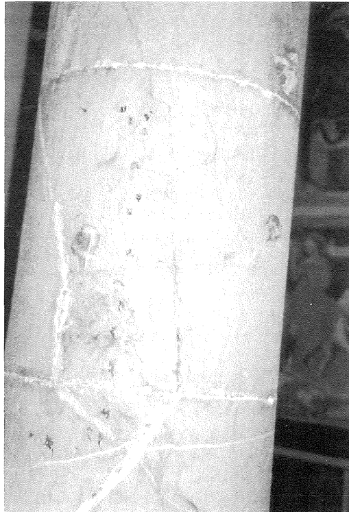
Fig. 3 – Particular of column 6
