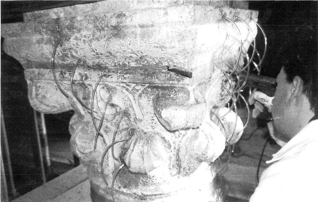
Fig. 6 – Consolidation of capital of column 6
