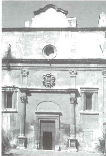
Fig. 3 – Image of the main façade of the church of Santa Maria dei Miracoli (XVI century) showing the different types of biocalcarenite (upper and lower orders) and the ocher film.
