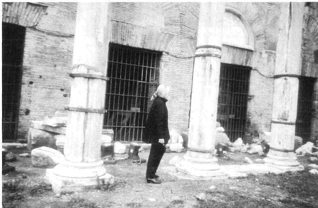
Photo 6 – Portico degli Dei Consenti . Shaft recomposed with overlapping drums of different height.
