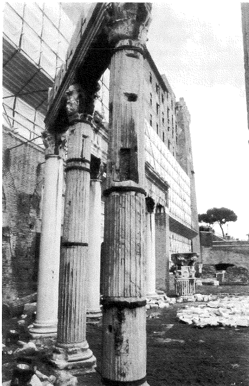
Photo 7 – Portico degli Dei Consenti . Grooves filled out by flat elements separated by wide listels.
