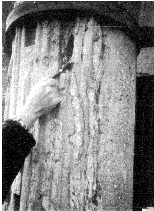
PHOTO 2 – Portico degli Dei Consenti . Column raised from ground; sampling point.
