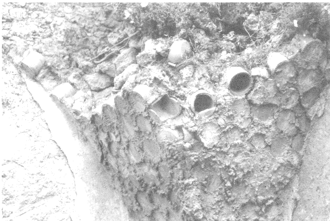
Fig. 3 – Arrangement of «caroselli» at arch impost of «Episcopio» in Gerace (circa 1700).
